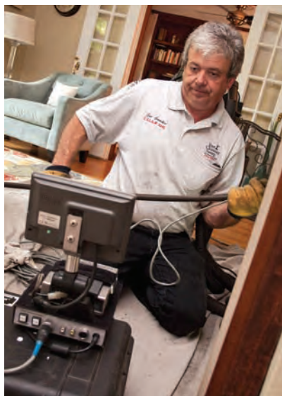
Photos by Brandon Smith | Joe Sauter of Your Chimney Sweep uses a special camera to inspect the flue liner of a chimney in an Indianapolis home.
